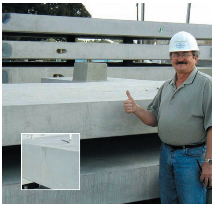
Finished precast units using Rheodynamic SCC
